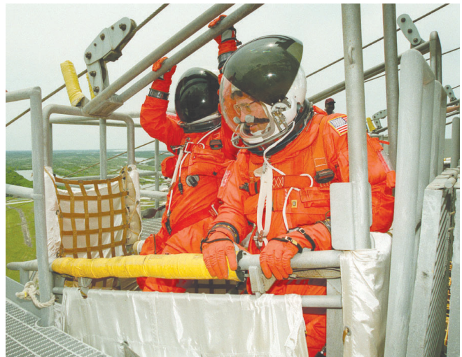
Astronauts climb into the slidewire basket on the Fixed Service Structure. The basket is part of the emergency egress system.
