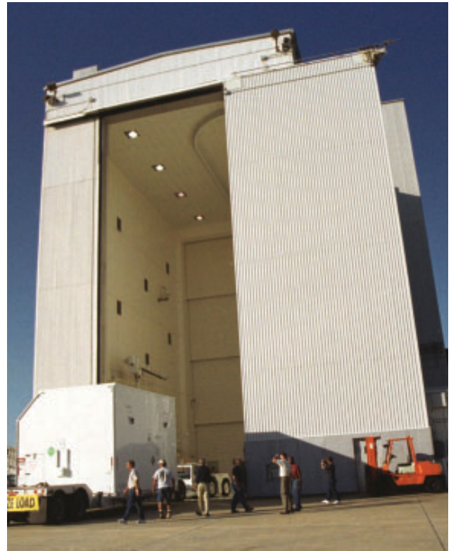
The truck delivering part of the equipment to be used on mission STS-109 moves into the Vertical Processing Facility at KSC.
