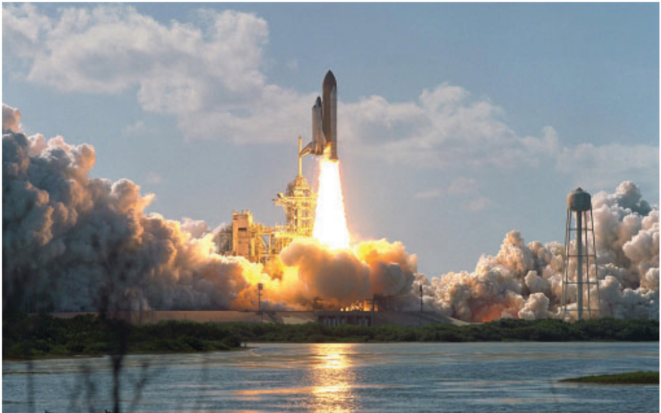
The 290-foot water tank at right of the launch pad holds 300,000 gallons of water that flow through outlets and flame deflectors in the Mobile Launcher Platform just before launch to act as sound suppression. The confluence of the water and intense heat and flames from the three main engines and solid rocket boosters creates the billowing steam seen (flowing left from the main engines and right from the boosters) during this launch of Space Shuttle Atlantis April 8, 2002, on mission STS-110.
