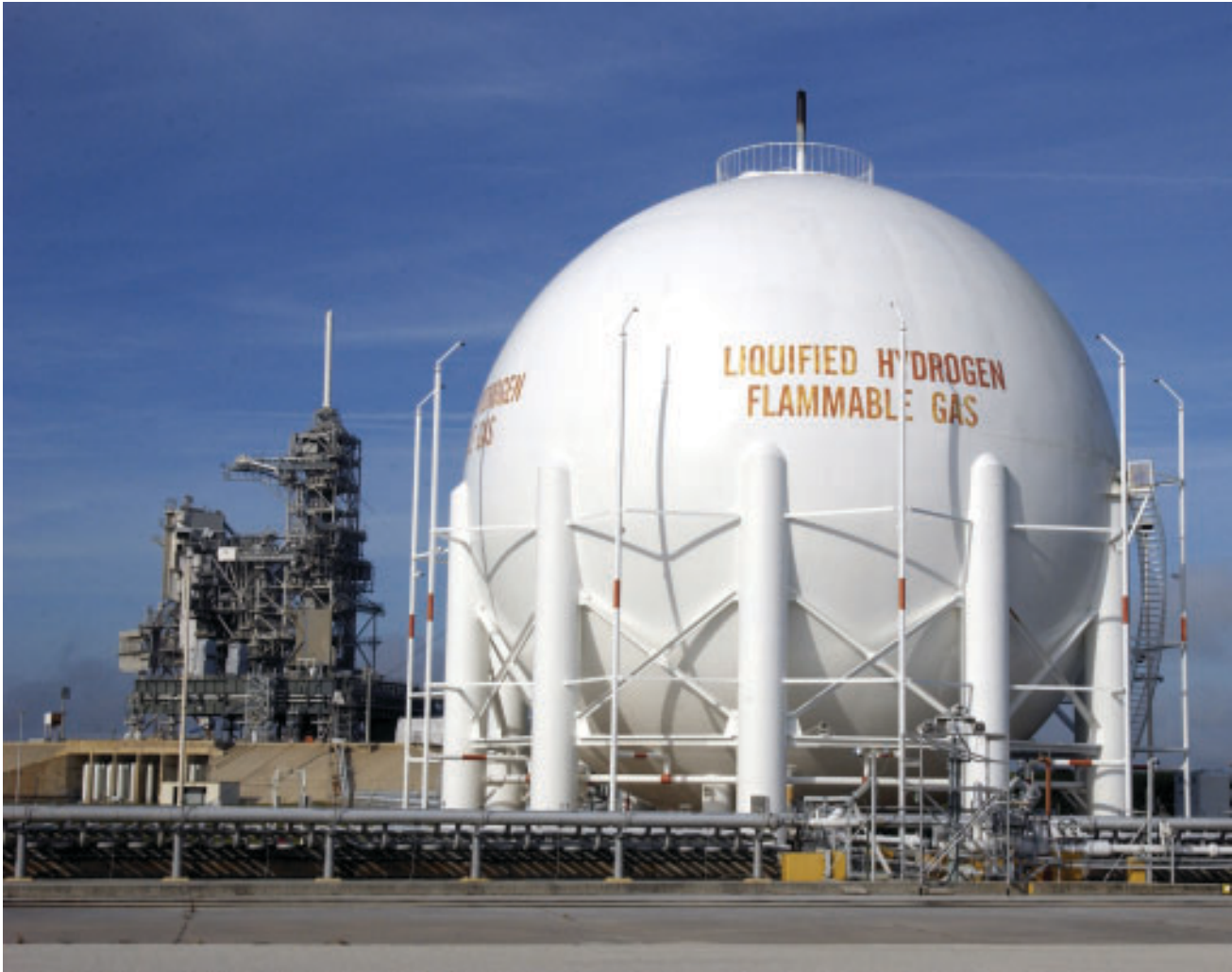
A large round tank that is actually a huge vacuum bottle stores the supercold liquid hydrogen at the launch pad. A similar round vessel holds the liquid oxygen. The liquid propellants flow to the orbiter's main engines.
