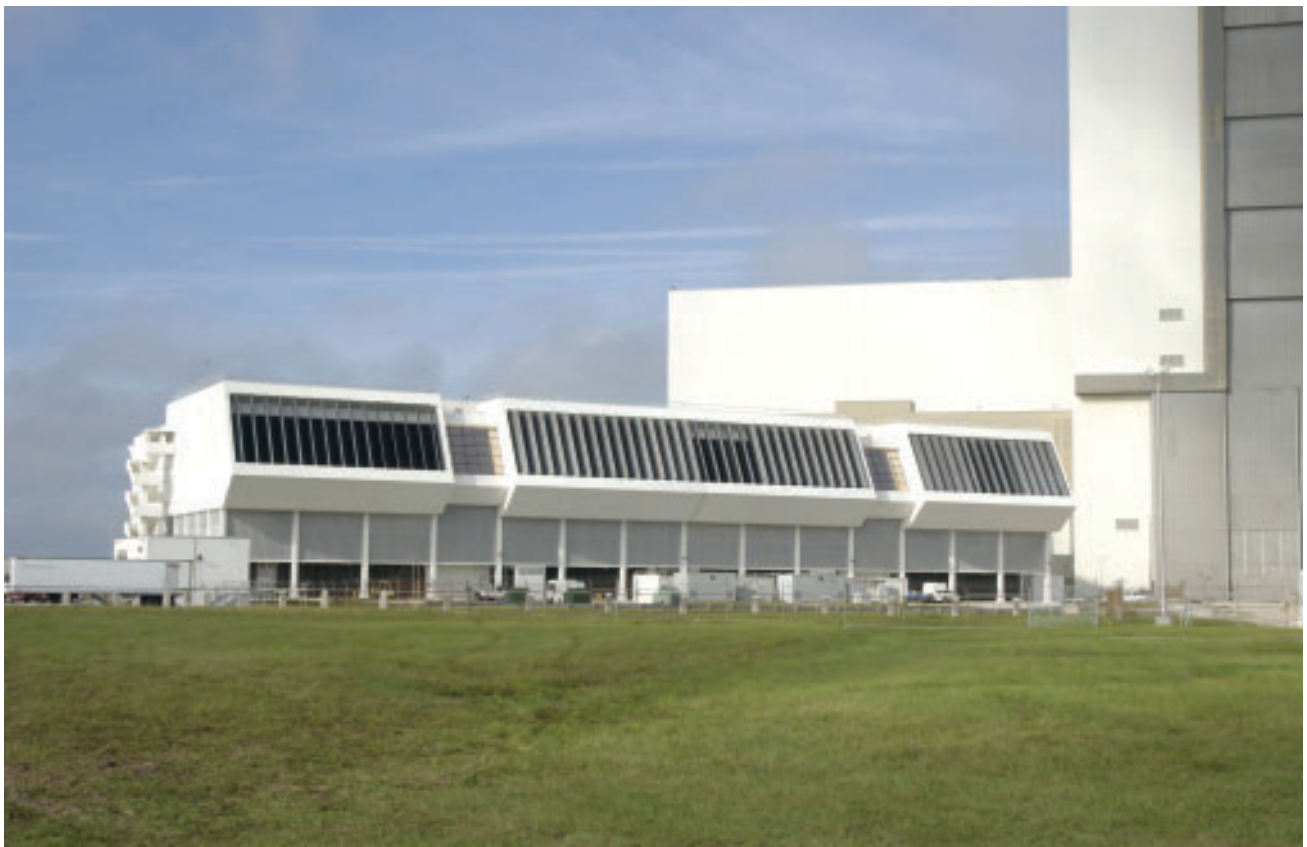
The Launch Control Center faces both launch pads.
