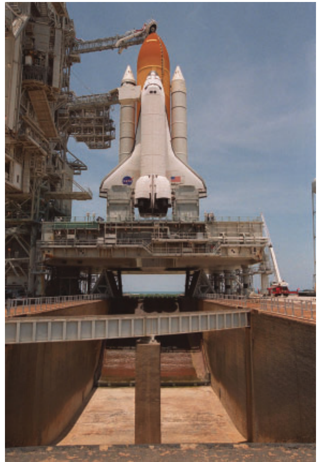
After rollback of the Rotating Service Structure, Space Shuttle Atlantis can be seen atop the mobile launcher platform (MLP) on Launch Pad 39A. Below the MLP is the flame trench, part of the flame deflector system that insulates pad structures from the intense heat of launch.
