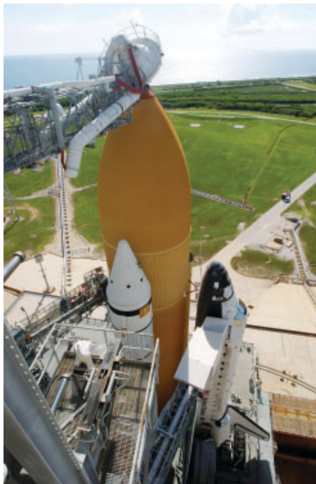
The gaseous oxygen vent hood (at top), known as the beanie cap, is located on the end of the highest swingarm attached to the Fixed Service Structure.
