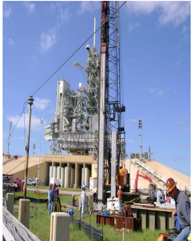
Workers install Lightning Protection System at Launch Complex 39B as modifications for Constellation continue
