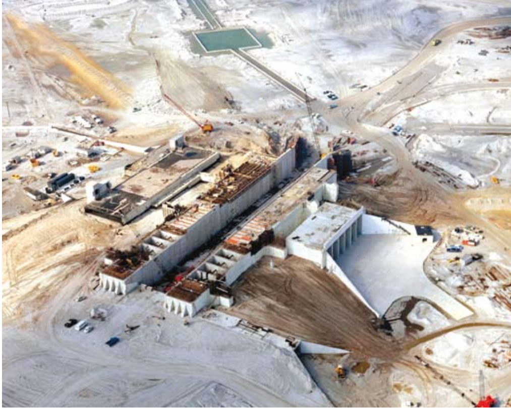
Construction of Pad A at Spaceport's Launch Complex 39. The pad hardstand contains 68,000 cubic yards of concrete.
