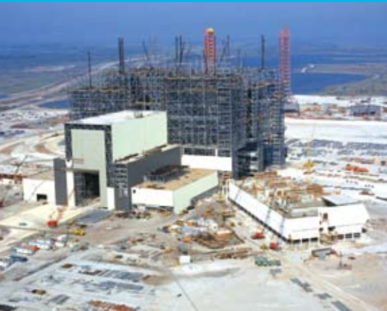
The steel framework of the Vehicle Assembly Building rises on Merritt Island during construction of America's Spaceport. The low structure at right is the Launch Control Center.
